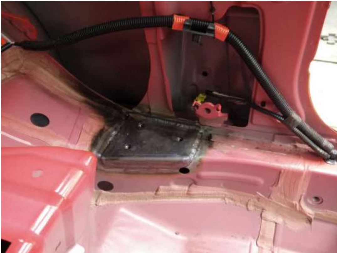
B pillar (middle of cage) foot plate.
